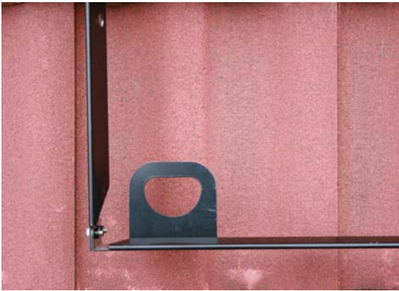
Fig. 15 - Loop in corner of frame
