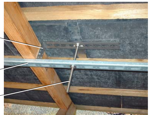
Fig. 23 - Channel and Rafter bracket
