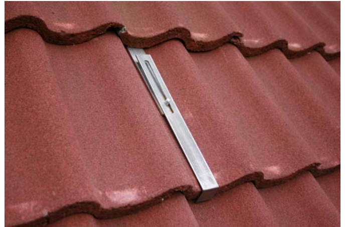
Fig. 12 - Additional support bracket (item 22)
