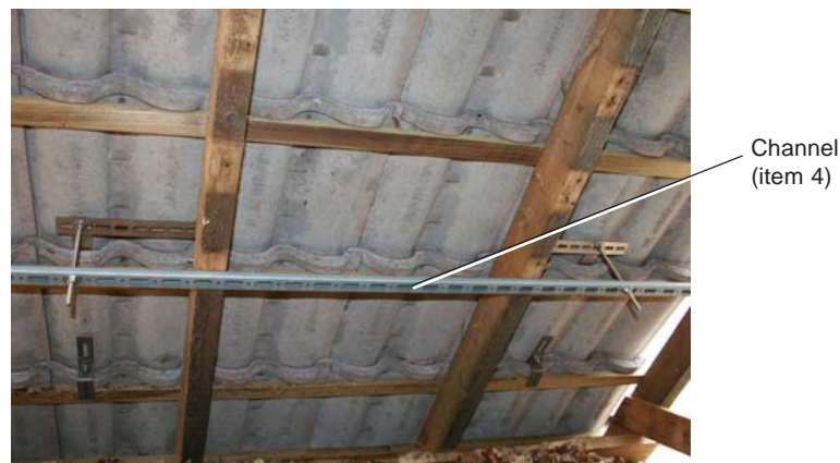
Fig. 10 - Channel and Rafter brackets
