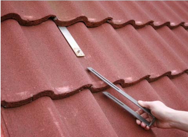
Fig. 11 - Additional support bracket (item 22)
